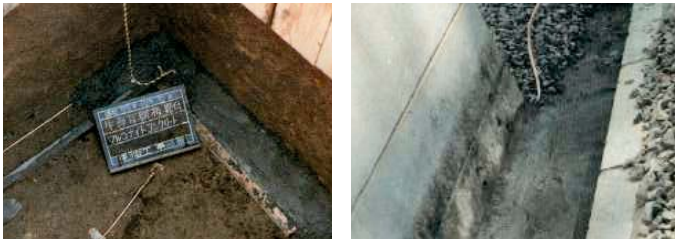
Laying SAN-EARTH M1C *One 25kg bag of M1C will cover approx. 3 meters (width 30cm)
