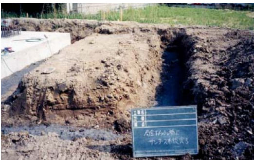
Laying SAN-EARTH M5C *One 25kg bag of M5C will cover approx. 3 meters (width 50cm) .
